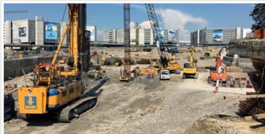
Geothermal activation of over 700 foundation piles
