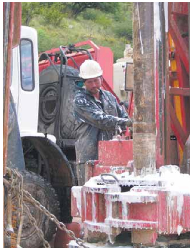
Foam circulation for down-hole hammer drilling in bedrock.
